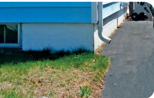
Roof runoff directed onto this driveway flows into the street and may be sending pollutants to a nearby waterbody.
